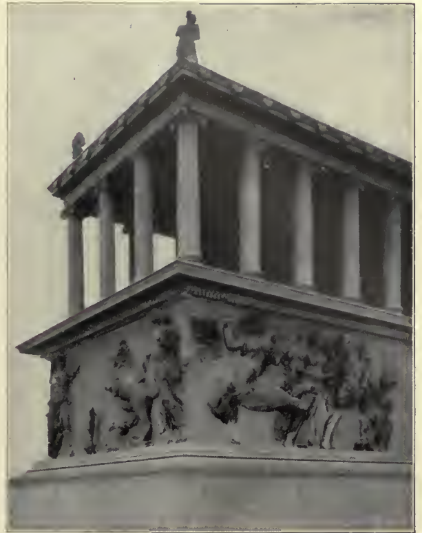
THE SOUTH WING, WEST AND SOUTH SIDES.
